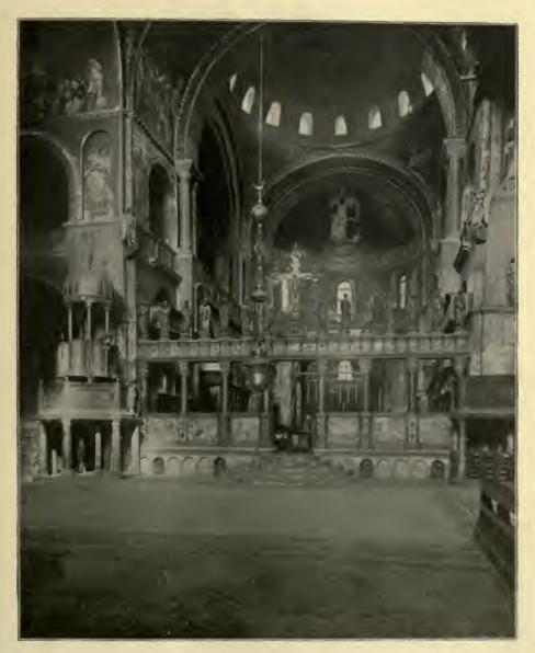
FIG. 4. NAVE OF S. MARK'S AT VENICE. Showing outward lean of the right pler.
